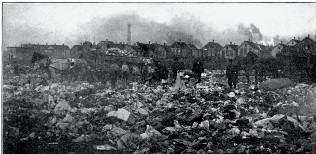
CITY GARBAGE DUMP IN THE CHICAGO STOCK YARD DISTRICT (RECENTLY ABANDONED).
